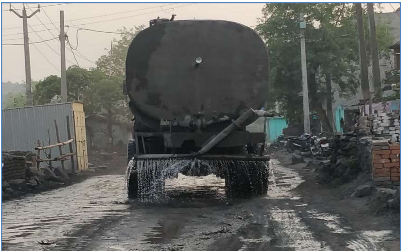
Water Sprinkling on Transportation Road
