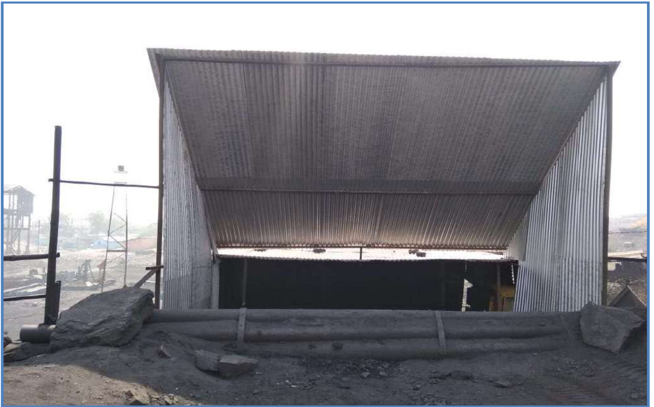
Picture 7 – Enclosed Coal Handling Plant
