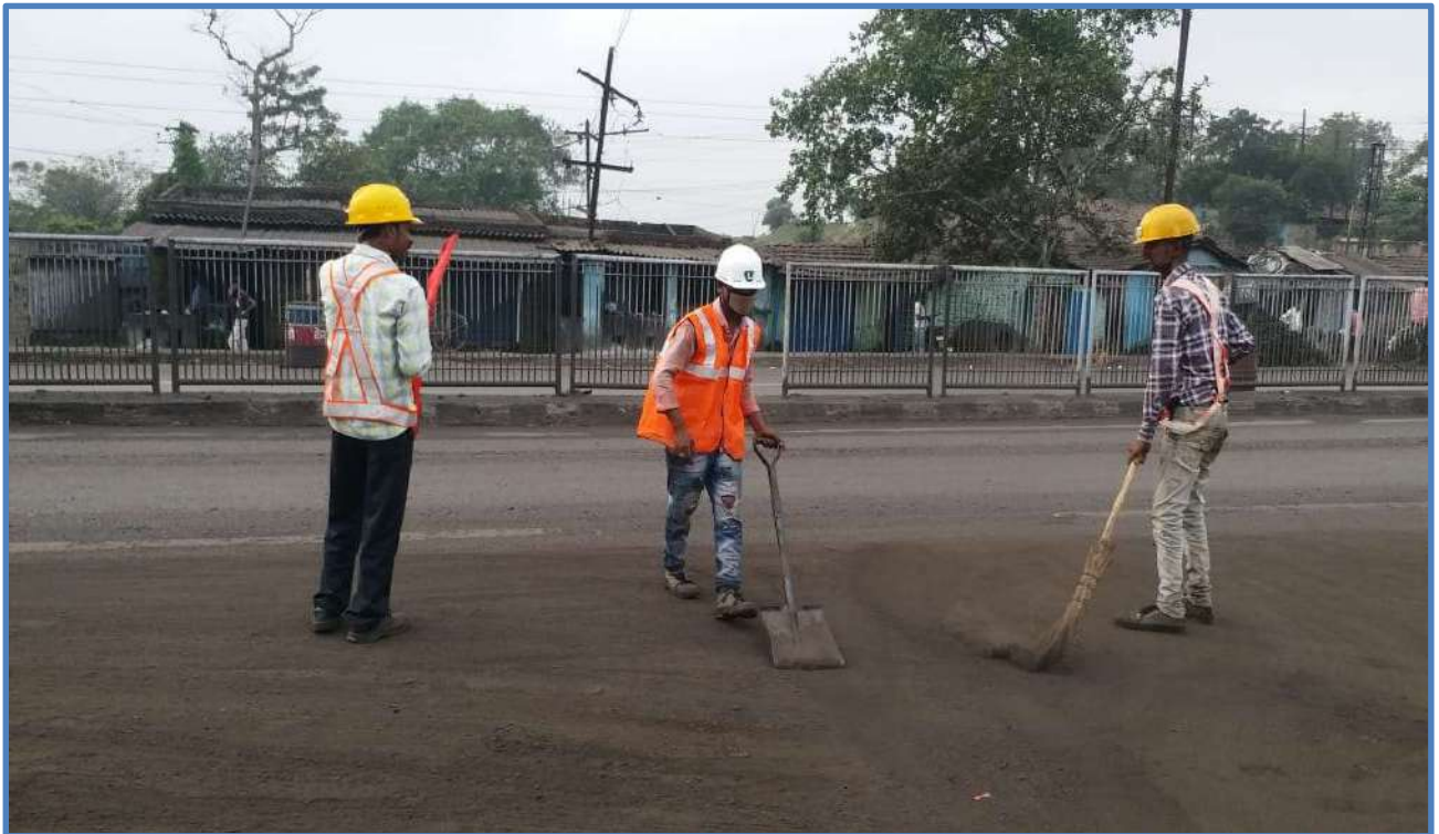
Picture 3 – Manual Sweeping of Public Road
